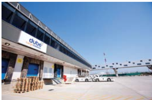
FIGURE 3: DUBE CARGO TERMINAL
